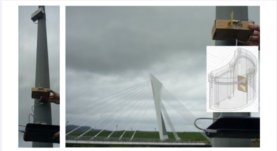
TILAS Project: Detail of the nodes with antennas and encapsulated customized deployment
